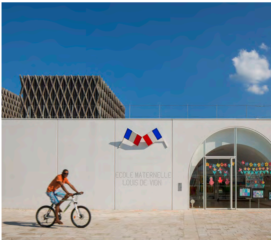
© AAVP – Atelier Architecture Vincent Parreira – Photographie Luc Boegly
